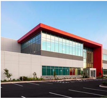
Data Centers New development, stabilized
