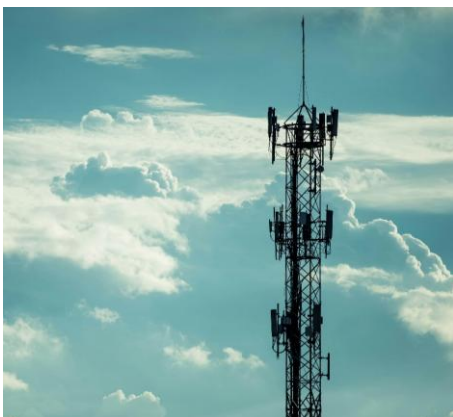
Digital Data center, cell towers, fiber
