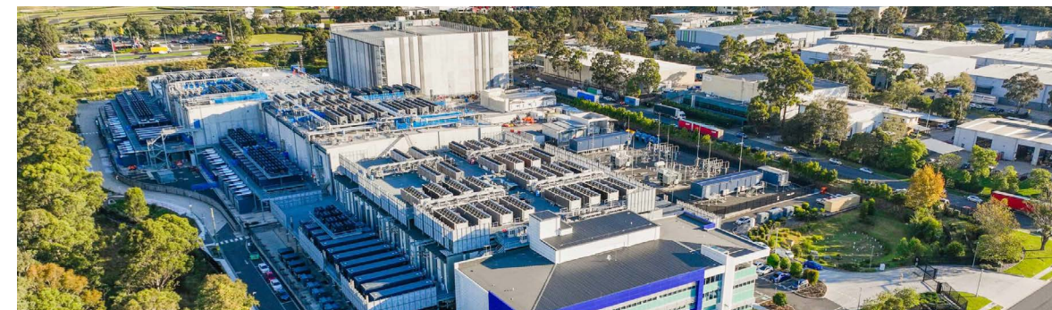
AirTrunk SYD1 data center located in Sydney, Australia
