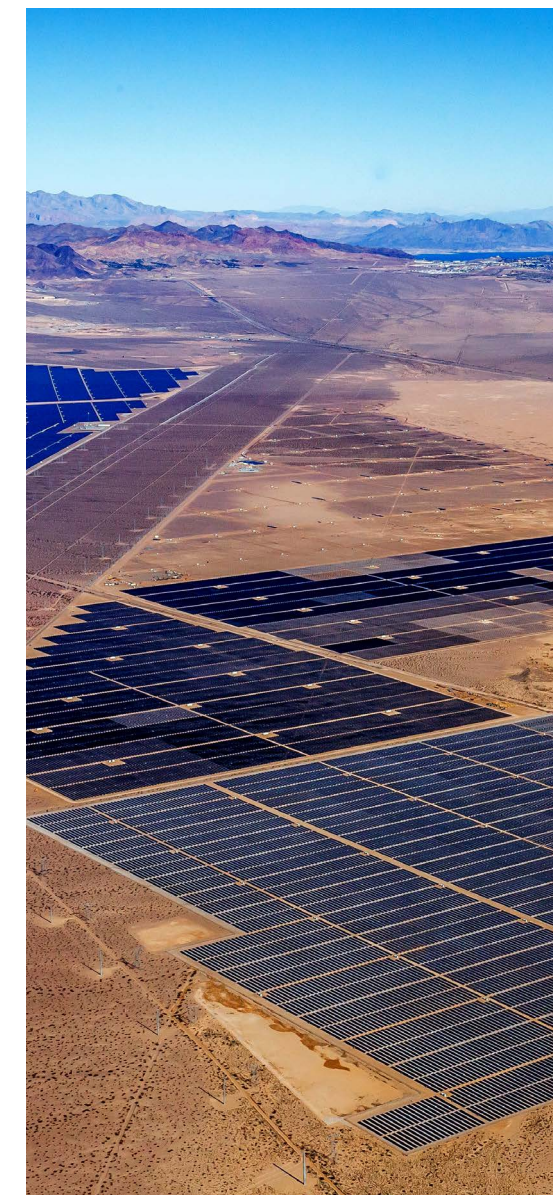
Westwood Professional Services Techren Solar installation near Boulder City, Nevada
